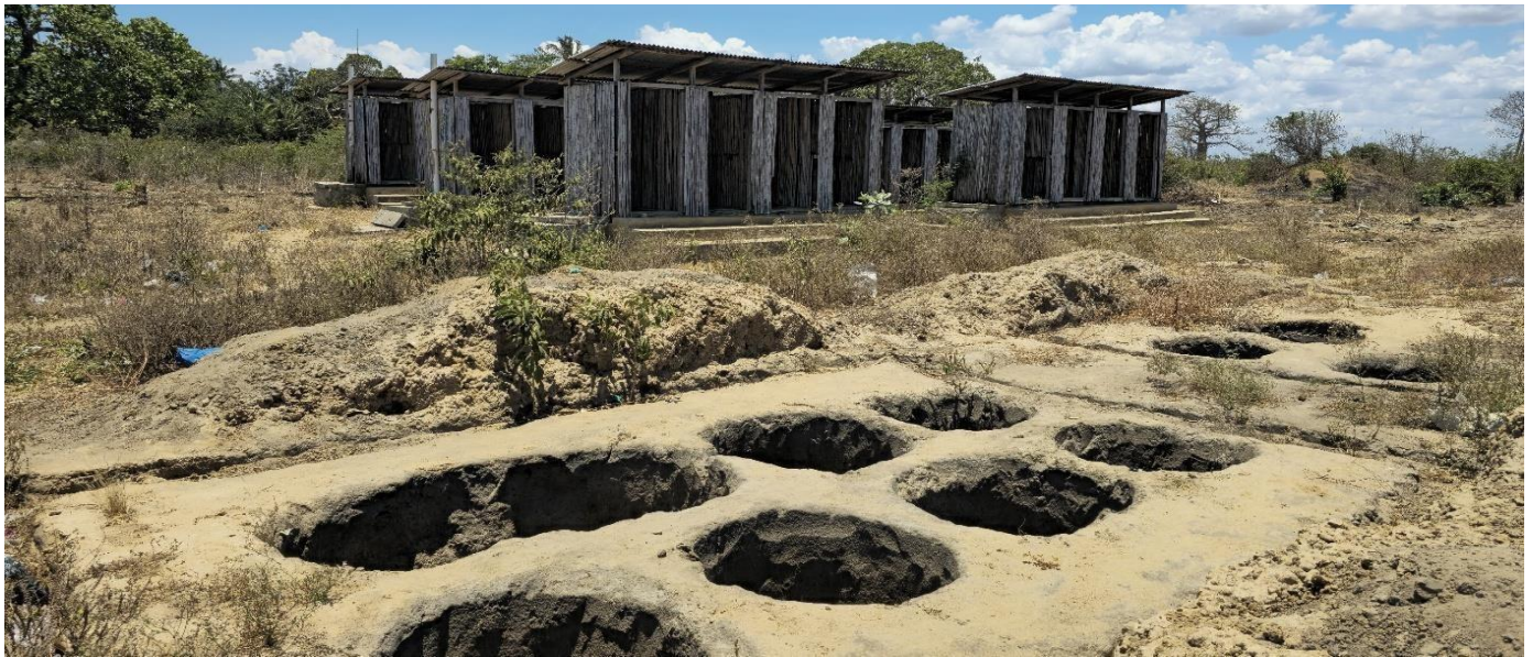
Figure 4.5: Abandoned latrine pits and filled pit latrines
