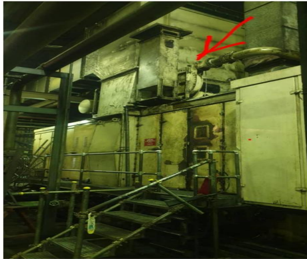
Figure 4: Exhaust frame blower
